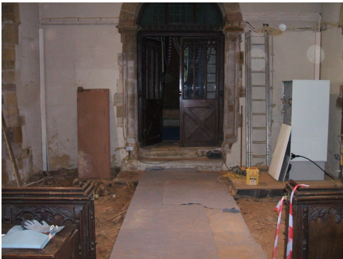
General view of the church interior during the lifting of timber flooring Fig 4
