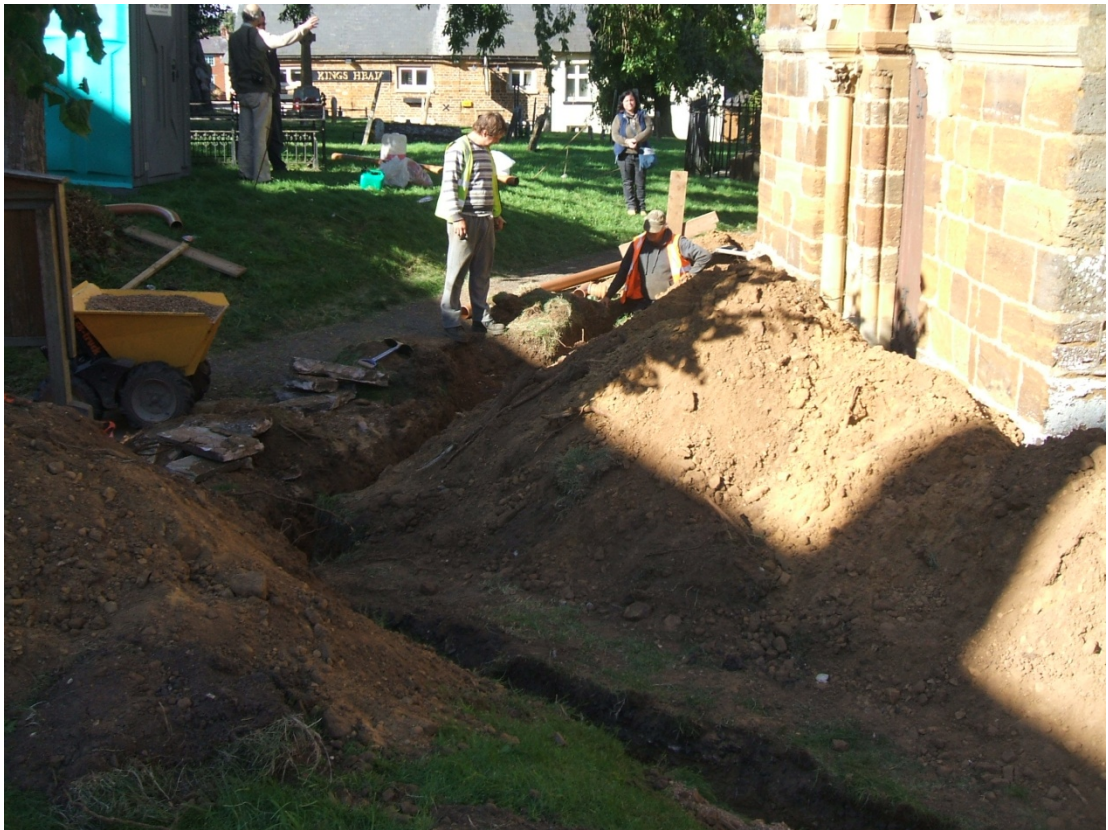
General view of the drainage trenches, looking north Fig 8
