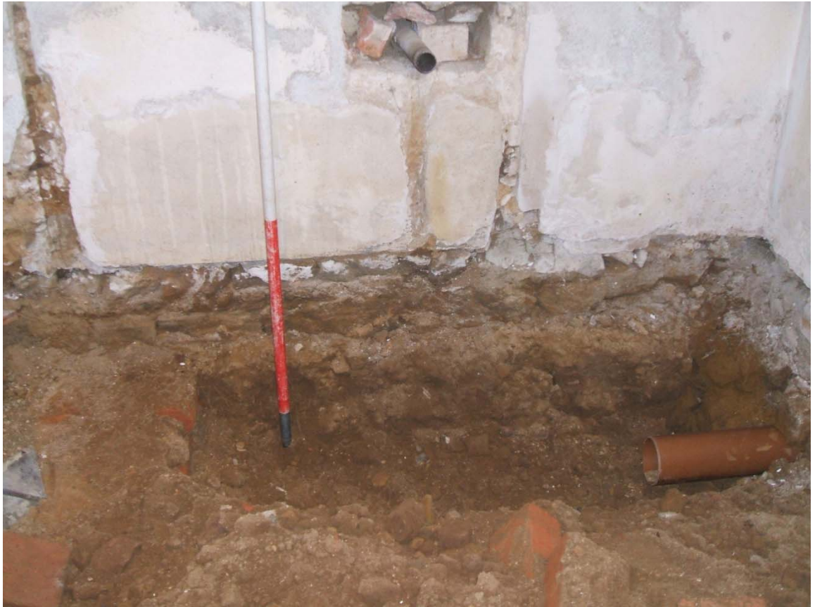
Laying the new drainage pipes Fig 6
