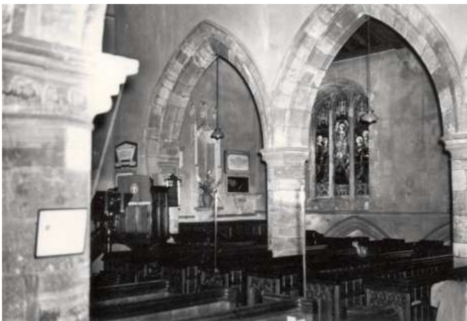
The two arch styles are seen in the photograph taken at the end of the nineteenth century:
