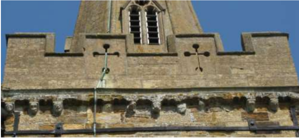
The 15 th century parapet
