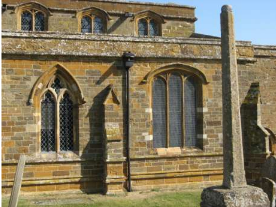
The exterior of the south aisle with the two different window styles
