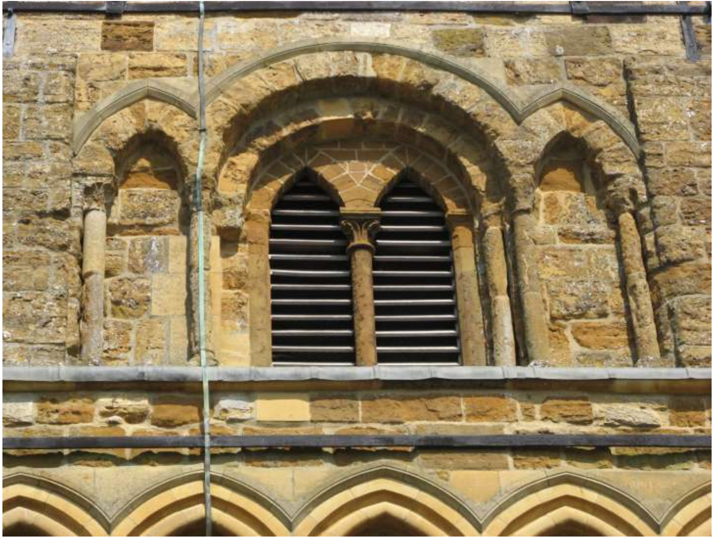
The third storey showing mixed Gothic and Romanesque arches
