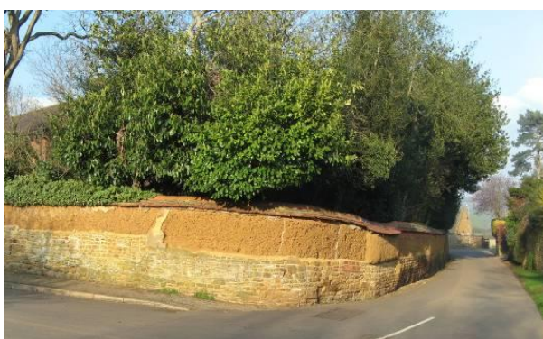
Cob wall at corner of Church and Holdenby Roads
