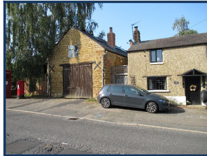
Figure 44 Former forge building in Brixworth Road
