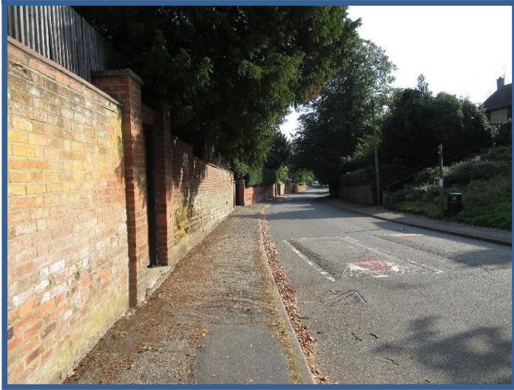
Figure 50: Brick walls in Church Road
