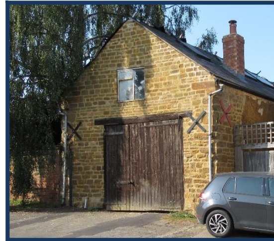
Figure 60: Wide doorway with timber lintel above at the Smithy, Brixworth Road
