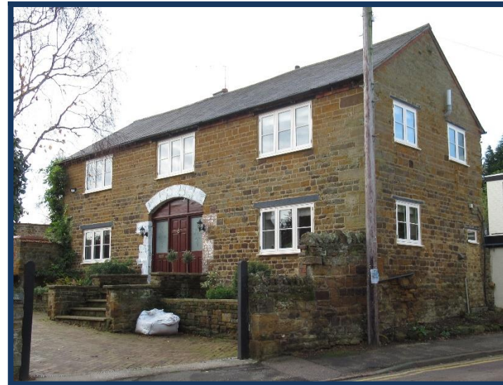
Figure 61: Arched doorway at former coach house, 6a Brixworth Road
