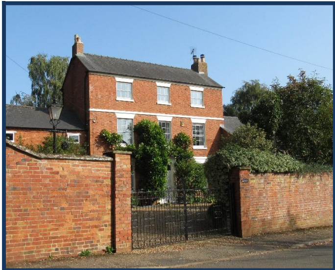
Figure 71: Holly House, 7 Church Road
