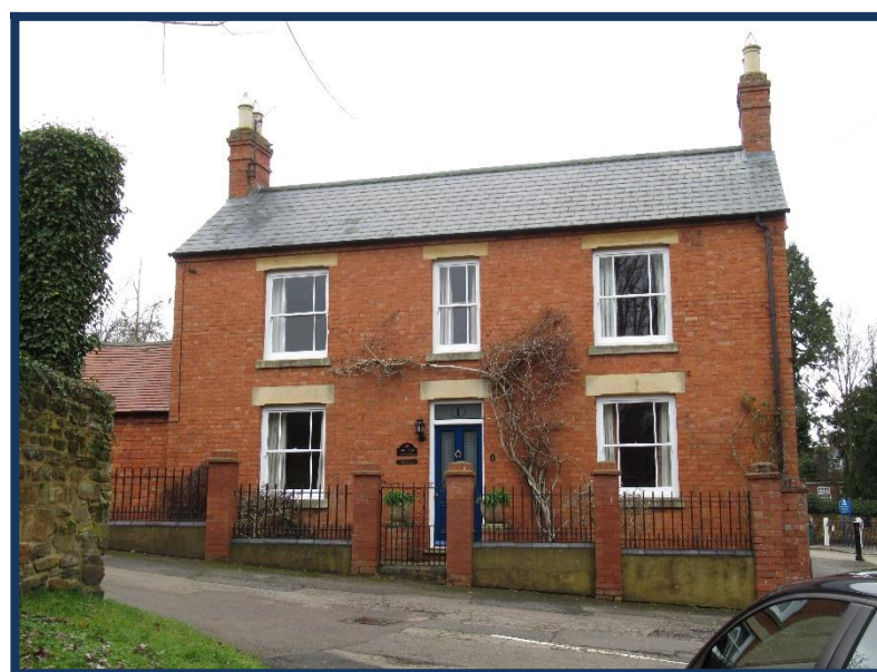
Figure 42: Vernacular buildings in Spratton, typical of materials, detailing and scale
