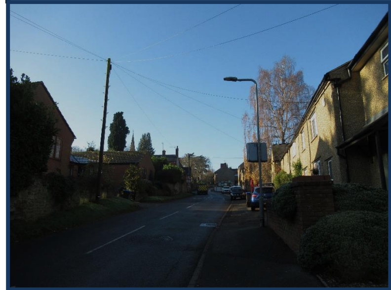
Figure 82: Telegraph pole and overhead wires in Brixworth Road
