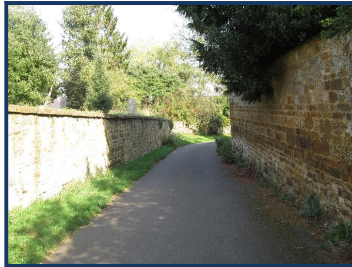
Figure 52: Tall ironstone walls either side of Church Lane
