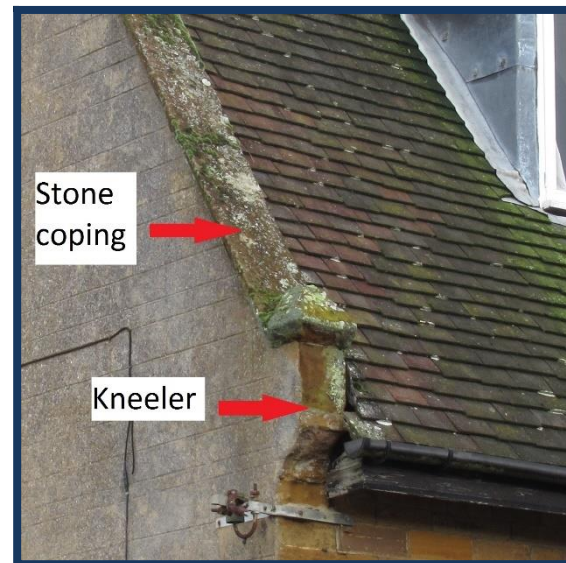
Figure 58: Stone coping on roof gable and stone kneeler at 14 Manor Road
