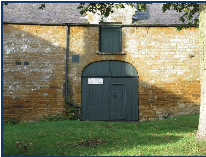
Figure 59: Arched doorway and opening above, the coach house at Spratton House
