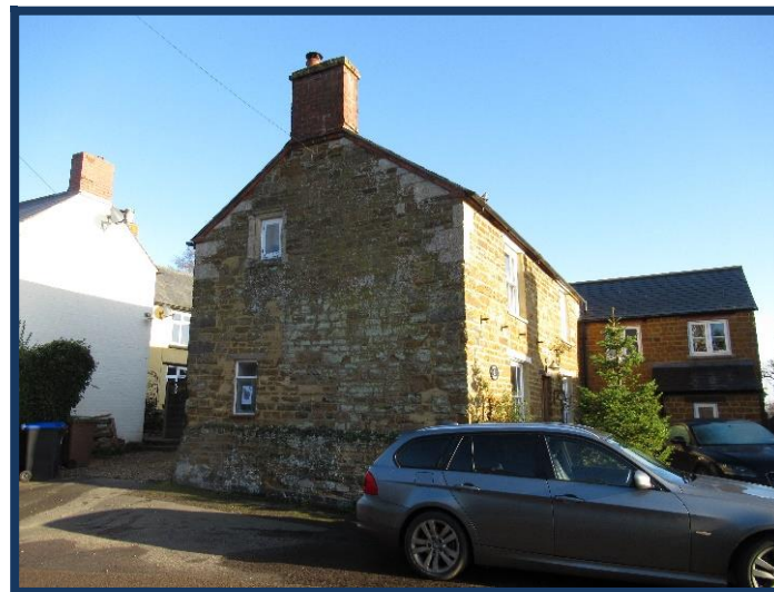
Figure 49: 24 High Street standing gable-end on to the street
