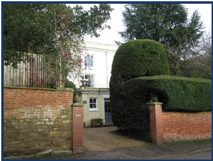
Figure 70: Spratton House, 5 Church Road
