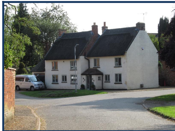
Figure 76 Radley House, The Walk
