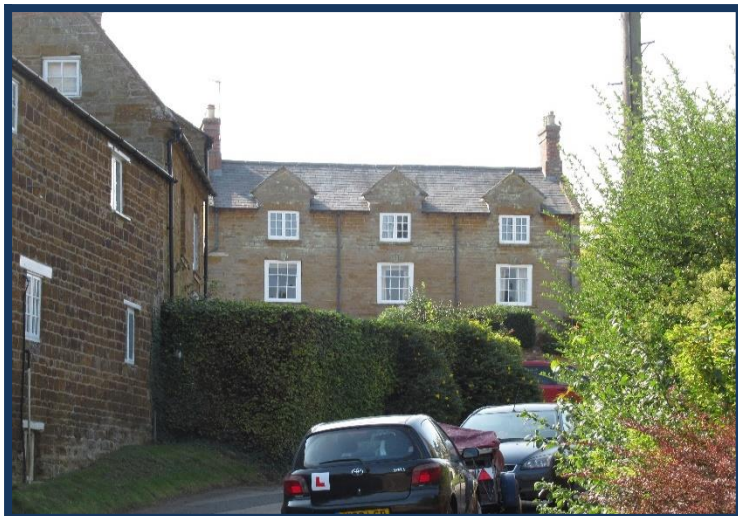
Figure 74: Manor House, Manor Road
