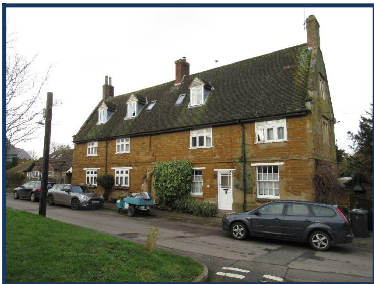
Figure 75: 14 and 16 Manor Road
