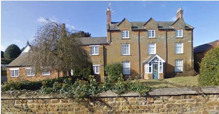
Examples of two story houses raised to a third level, Manor in Manor Road, early 19C, and Olde White Horse, early 20C
